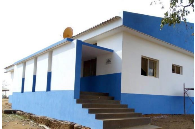
Figure 10. The newly renovated Mirate village clinic. Battery Minerals has reinstated electricity, painted the clinic inside and provided new fixtures and linen.
