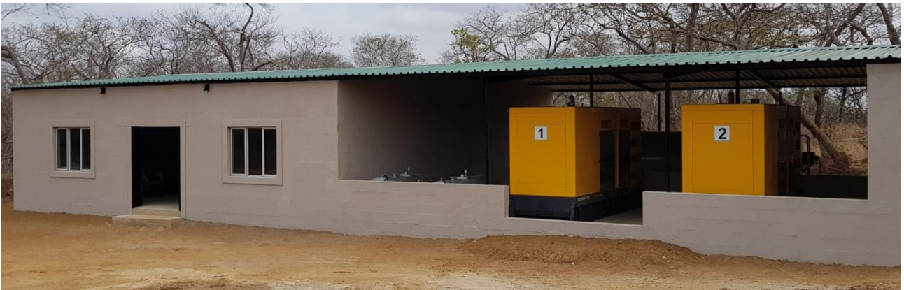
Figure 3. Montepuez Graphite Project: View of workshop, power generators and fuel storage at the permanent camp.
