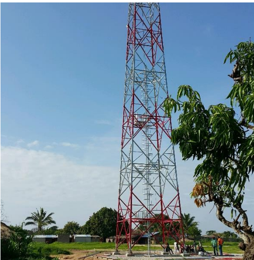
Figure 11. Communications tower installed by provider for benefit of Battery Minerals and surrounding communities
