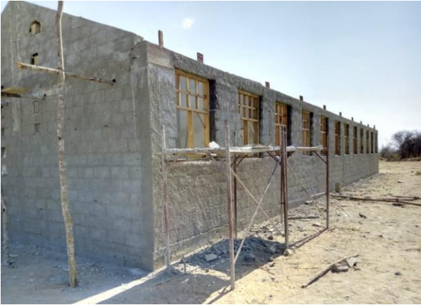
Figure 9. Construction status of new school at Nkawene village
