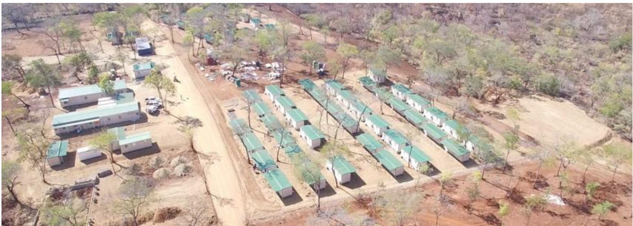
Figure 1. Montepuez Graphite Project: Aerial view of camp. The camp is due to receive the first residents in November and will accommodate up to 100 people
