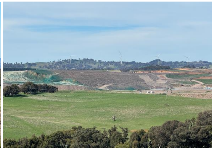
Figure 14. Cadia's tailings dam
